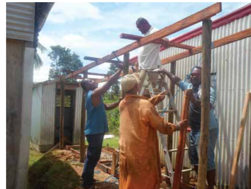
Constructing the undercover walkway from the kindergarten to the toilet block.
